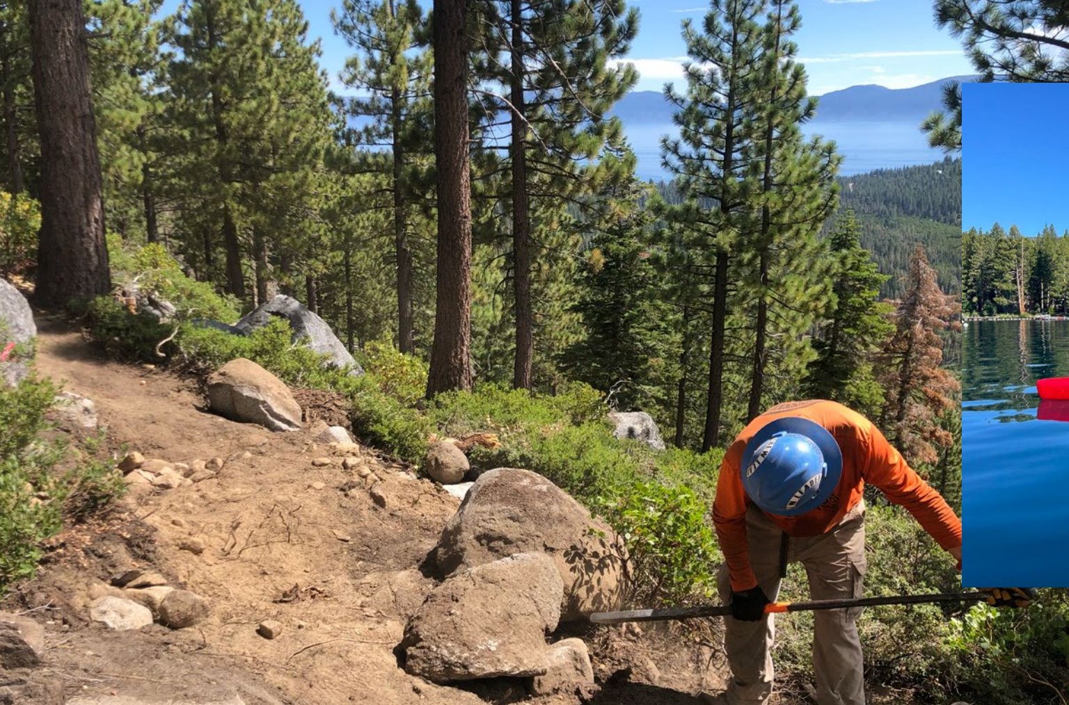
TAMBA Trail Work on Meeks Ridge Trail
